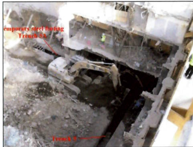
Figure 23 Overview of steel footing trench
