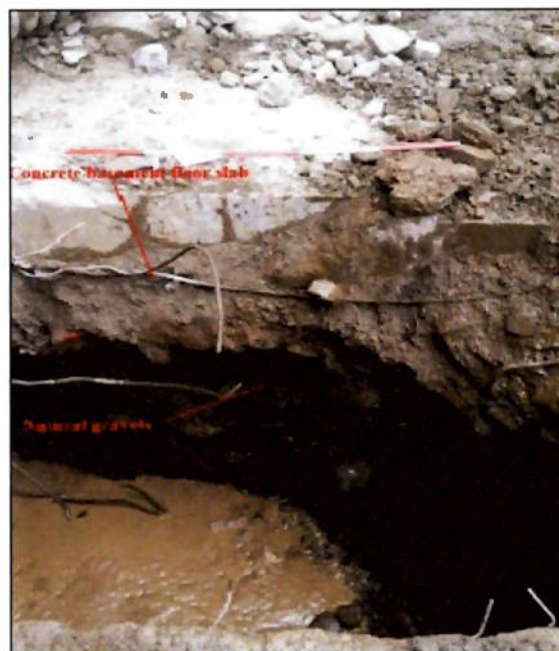
Figure 25 Trench B, concrete and natural gravels
