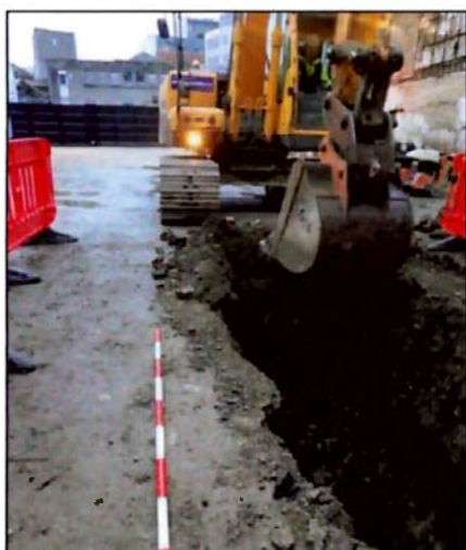
Figure 45 Trench 1, from the east
