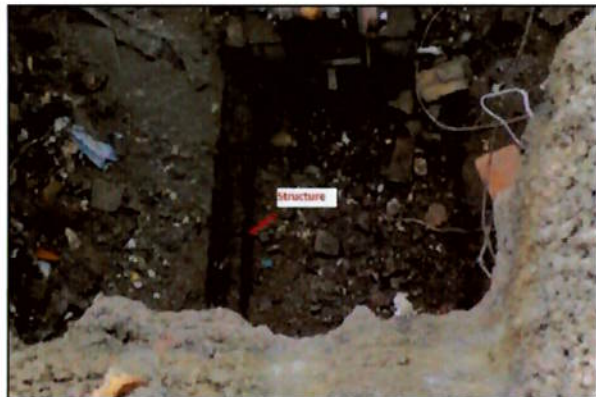
Figure 58 Foundation from the east
