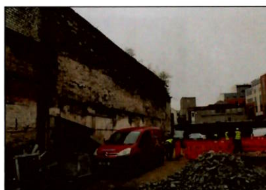
Figure 94 Building 4 from the east
