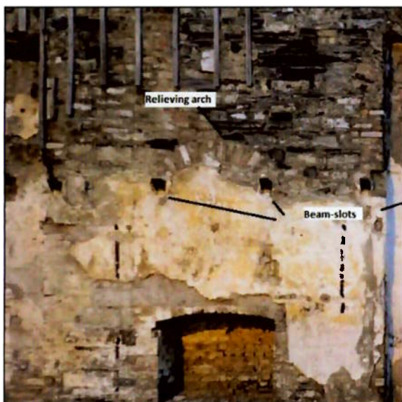
Figure 78 The relieving arch and beam-slots
