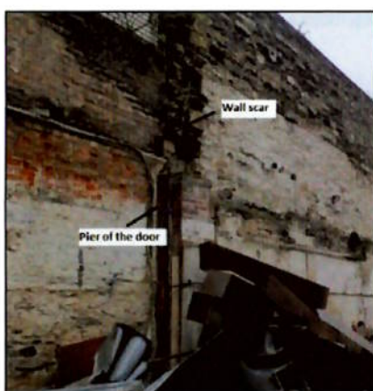
Figure 95 The door pier
