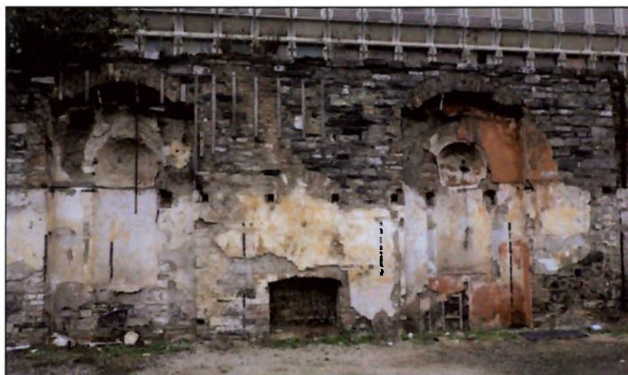
Figure 74 Building 2, from the south
