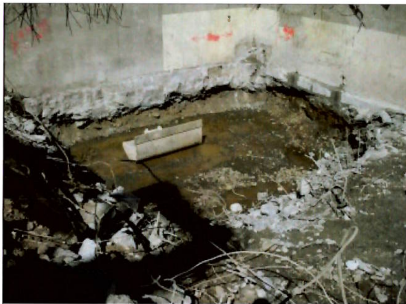
Figure 27 Trench 4, temporary crane base
