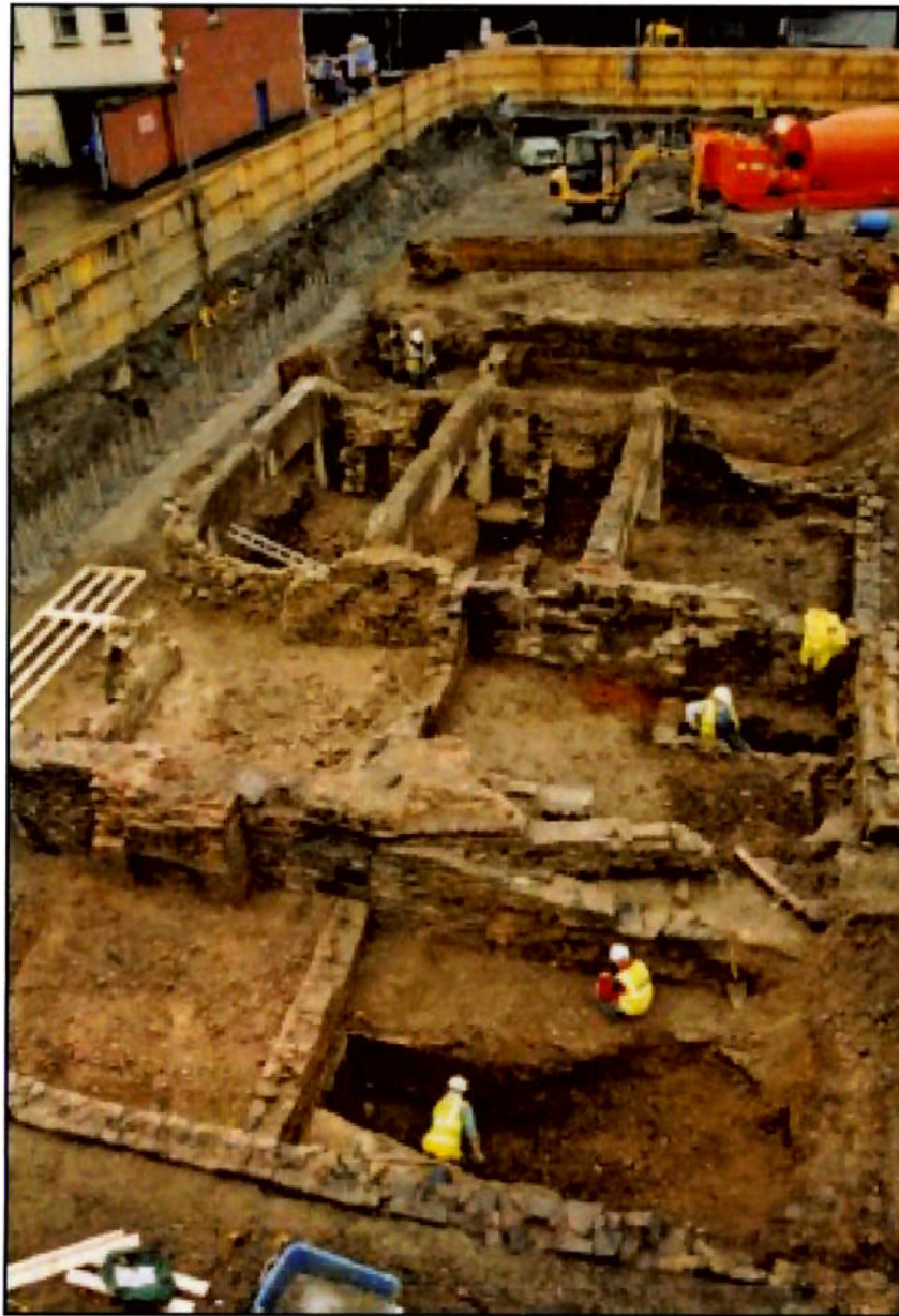
Figure 100 Nos 58-66 Parnell Street/Moore Lane, structural remains
