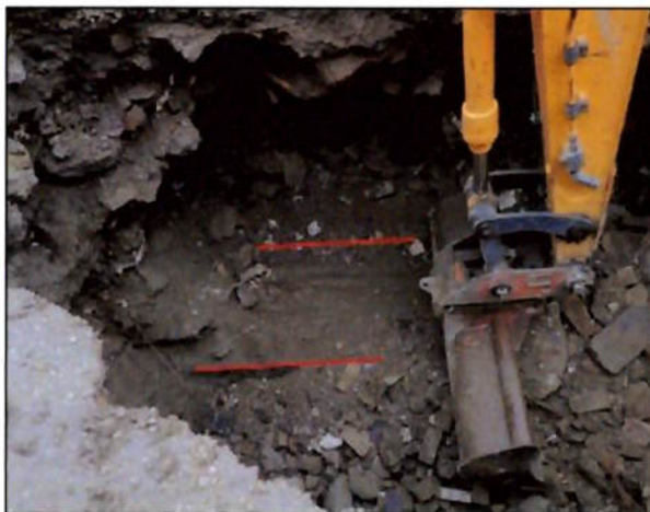
Figure 60 The structure from the north
